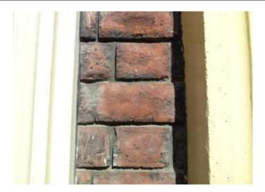
Brickwork with paint/render/ceramic tiles removed, note the raked joints. These are unlikely to have been an original feature of the building's exterior. Image: WCC DSC01921, July 2011.
