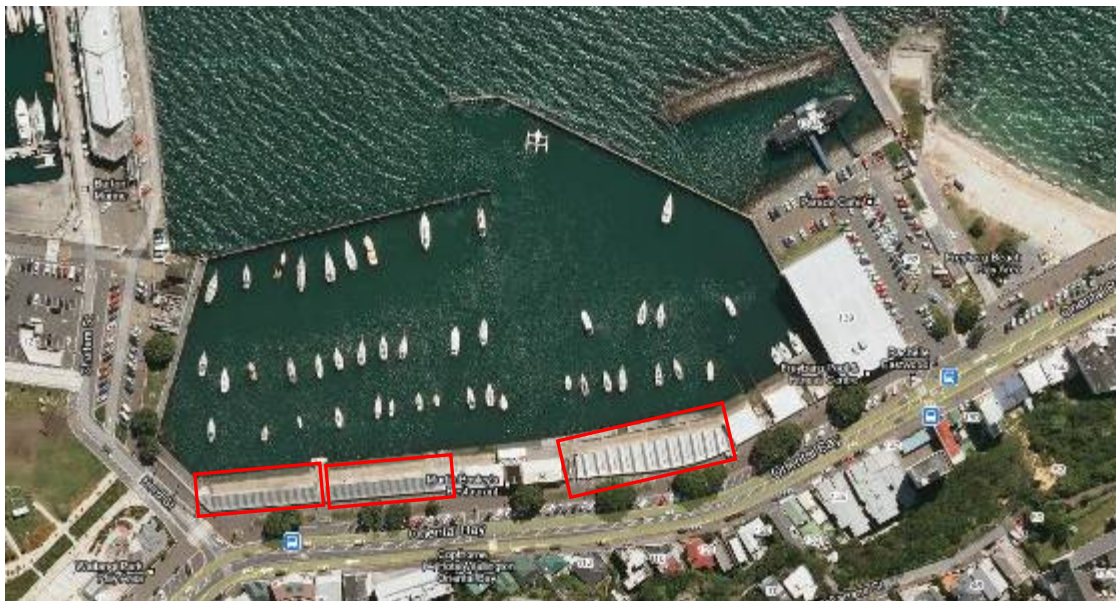
Aerial view of the boat sheds. From left to right: sheds 1, 2-13, 14-27, 38-49 (Image: Google Maps)
