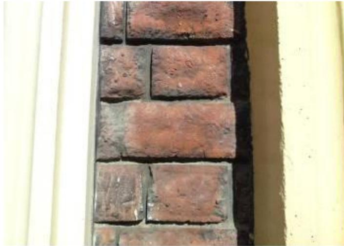
Brickwork with paint/render/ceramic tiles removed, note the raked joints. These are unlikely to have been an original feature of the building's exterior. Image: WCC DSC01921, July 2011.
